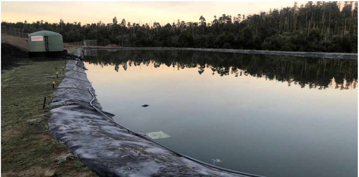
C-Cell Leachate Balancing Pond (SS9)
