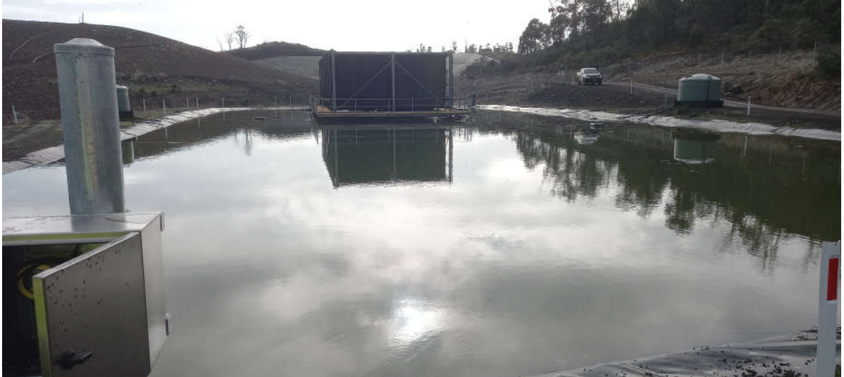
C-Cell Main Leachate Pond (SS10)
