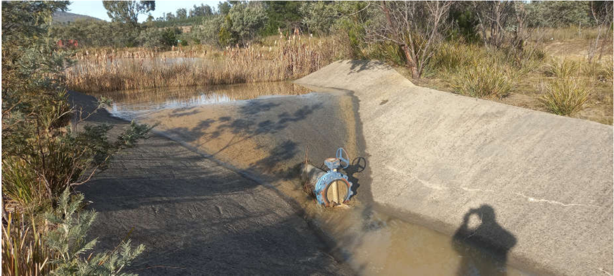
(B-Cell Primary Stormwater Pond SS3)
