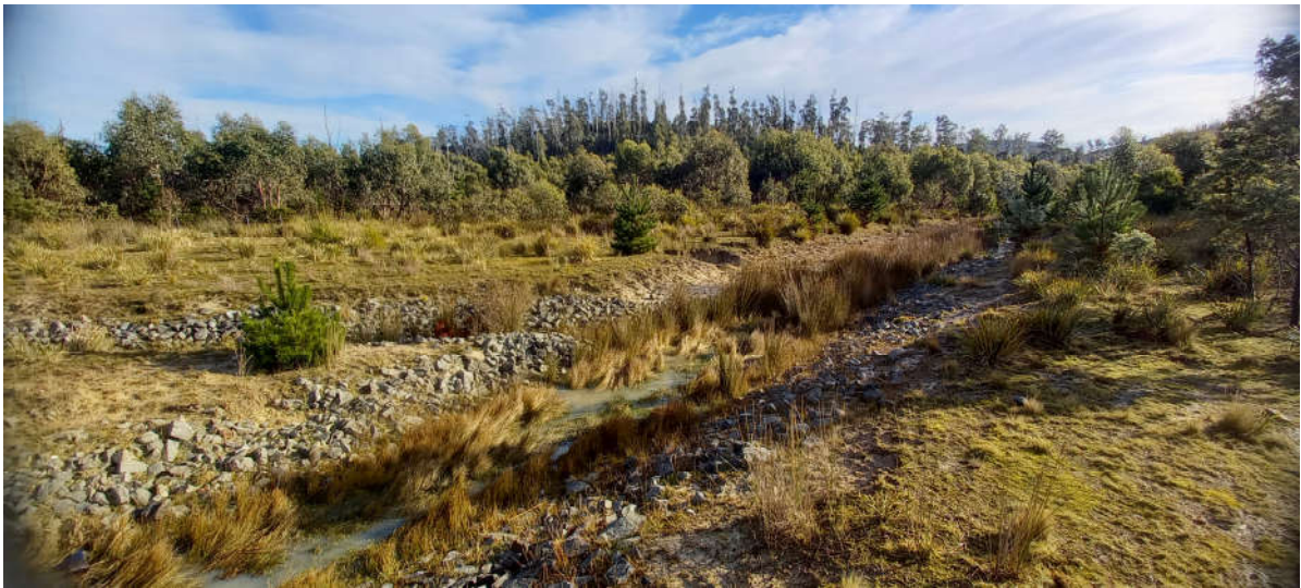
Primary Stormwater Pond Drain Towards (SS5)
