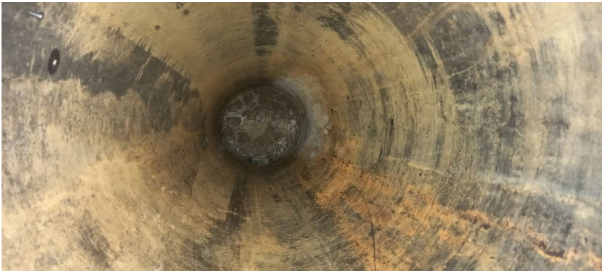
C-Cell Main Leachate BP Seepage Pit (SS8)
