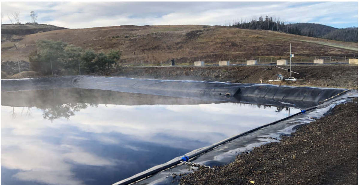
B-Cell Primary Leachate Pond (SS1)
