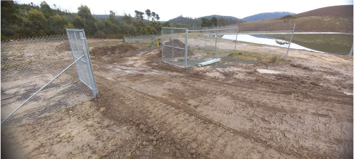
Impassable Vehicle Access Road to BH13
