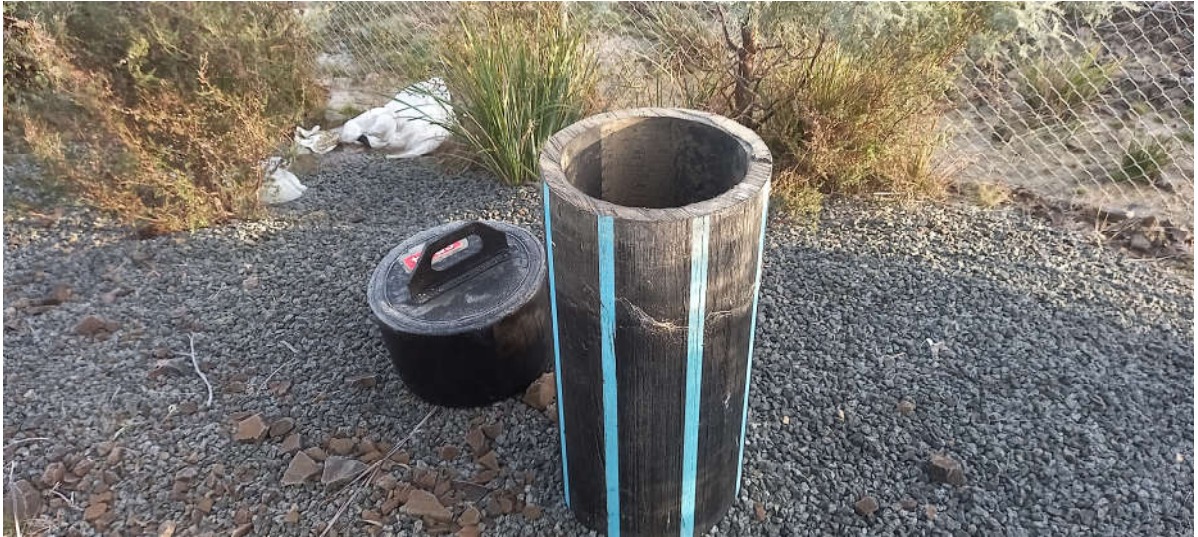
C-Cell Main Leachate BP Seepage Pit (SS8)
